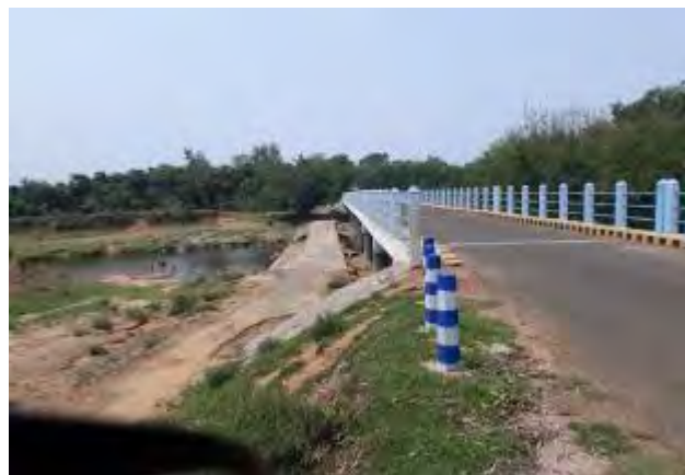
Access Bridge crossing on Arkasa River at Ahanda Ghat
